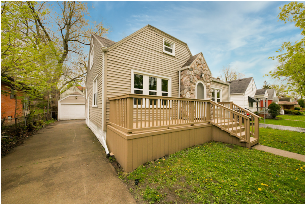
Panel B: After rehabilitation
